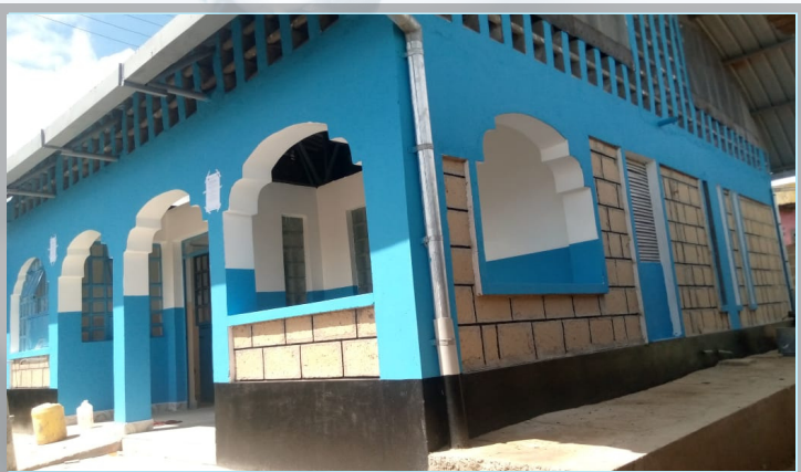
Ihindu Public Sanitation Facility
